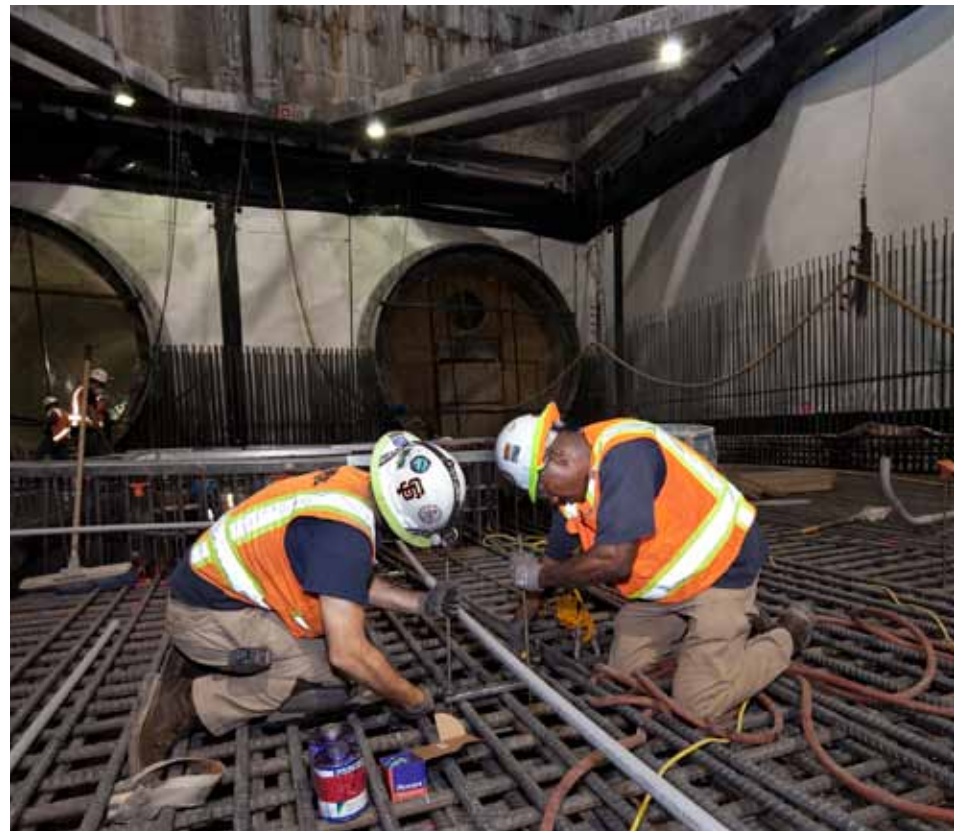
Apprentice Marlon Anderson, right, with Andrew Ammsso of Local 441.
