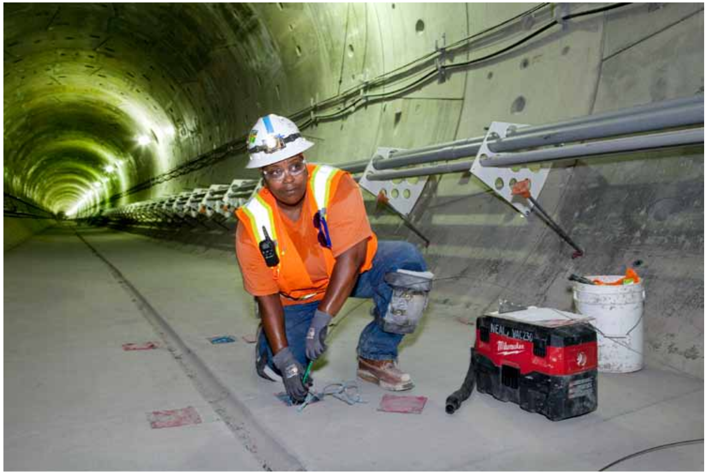
Quiontessa Riddick pulling wires in the tunnel under the MLK station.
